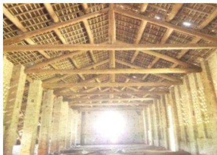
Figure 24. First floor of the central aisle
