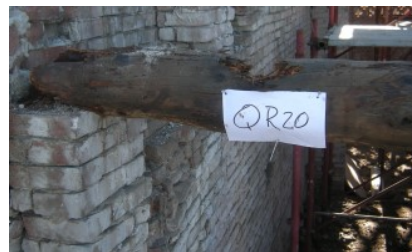
Figure 32. Local damages and deterioration on supports of timber elements.
