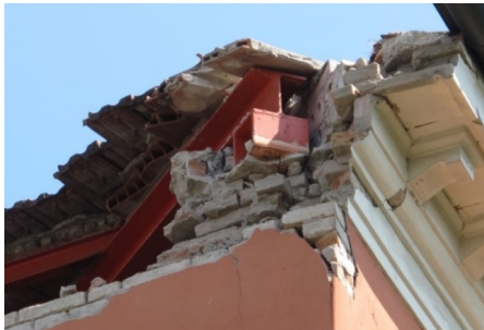
Figure 3. 2012 Emilia earthquake - Collapse due to a wrong intervention, without the realization of an upper curb on the masonry wall to distribute the horizontal forces transmitted by the new steel beams
