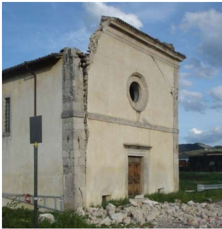
Figure 6. 2009 L'Aquila earthquake - wall detachment due to the absence of a roof structure capable of ensuring a box-like behavior of the church
