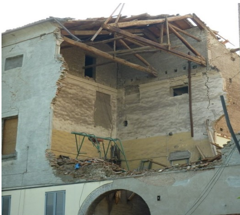
Figure 1. 2012 Emilia earthquake - Collapse of external slender walls due to the absence of the intermediate floor and insufficient stiffness at the roof level.
