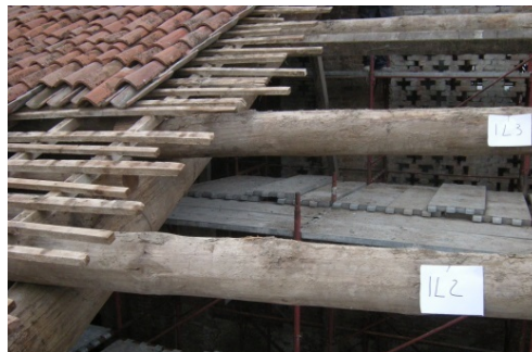
Figure 26. Flexible timber roof of the barn.
